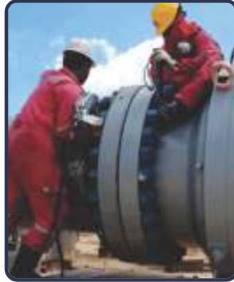
Bolt Torquing & Tensioning
