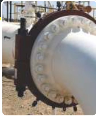
Leak Sealing & Live Repair
