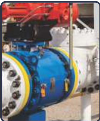
Valve Flushing & Lubrication
