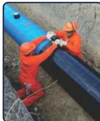
Anti Corrosion Coating
