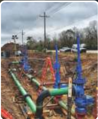
Hot Tapping & Line Stopping
