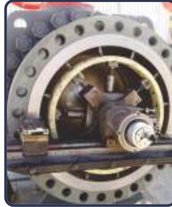
Onsite Machining & Cold Cutting
